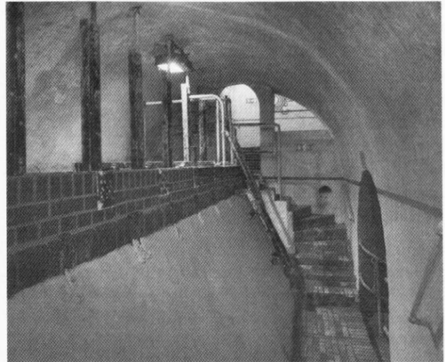
Overflow weir under the Albion Hotel.
